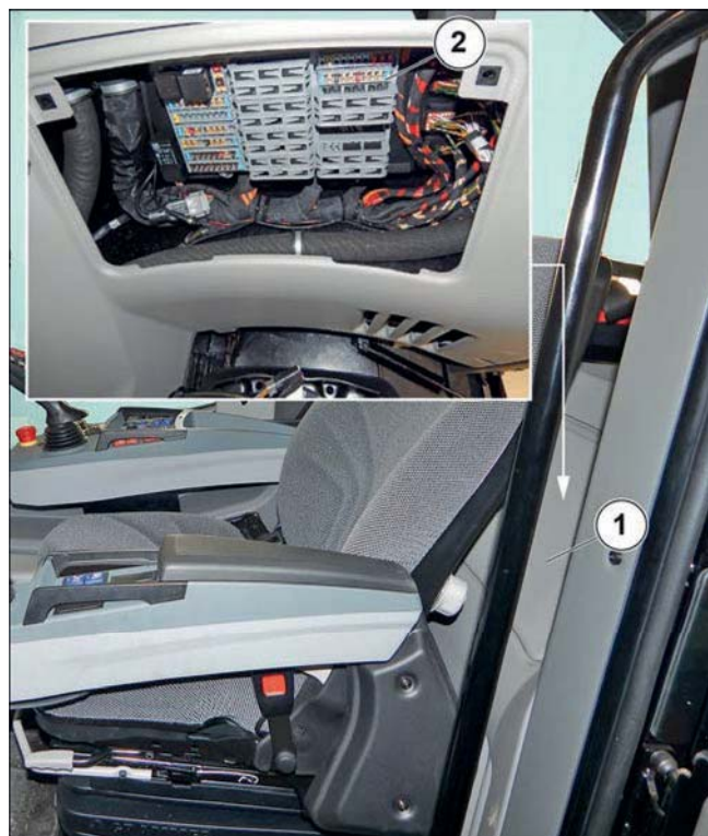
Figura 200: Fuse and relay in cab
